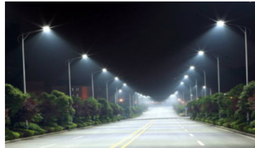
50,000 street lights and 6000 sign lights
